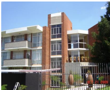
View of Complex
